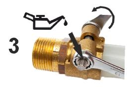
3) Put the tightening bolt on it's place and start tightening it with proper tools. Bolt thread is pre-lubricated in a factory but in case of long storaging time or other conditions like wetness some extra lubrication like vaselin may be added in attend to avoid threads cold welding. Use lubricant that is especially made for thread lubrication and do not put the lubricant on the pipe.
